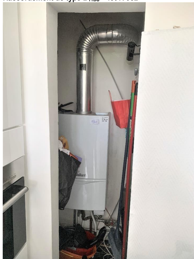
Raccordement de type B 11BS – lot R 082
