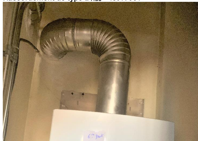
Raccordement de type B 11 BS – lot R 061
