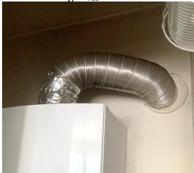
Raccordement de type B 1BS non conforme – lot R 022
