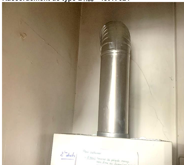
Raccordement de type B 11BS – lot R 021
