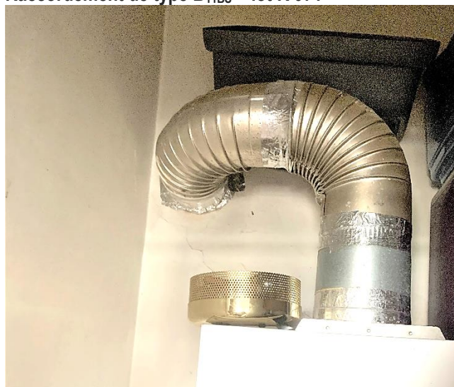
Raccordement de type B 11BS – lot R 071
