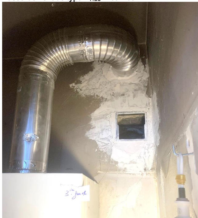
Raccordement de type B 11 BS – lot R 032
