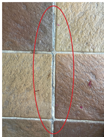
Fissuration des joints
